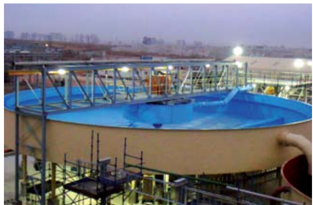
The 26 m diameter thickener at GBG's Burnstone mine.
